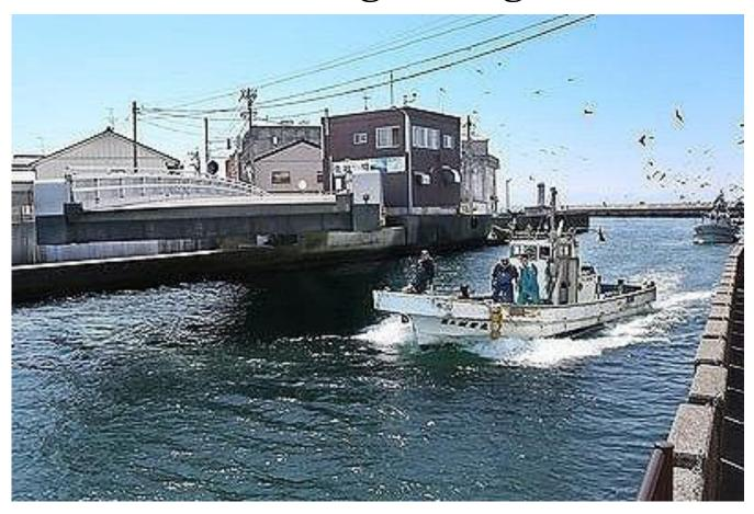
Ikuji Naka-bashi is a moving bridge made in 1982. This bridge was made to expand the Kurobe Fishing Port area. It is located in Aimono-cho in the area of Ikuji. Ikuji Naka-bashi rotates to allow boats to pass through. This is one of the most unique bridge in the world. (Seimei J.H.S.)
